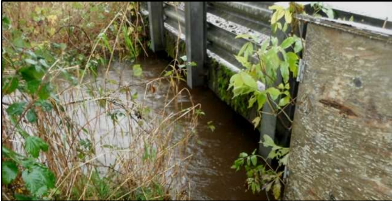
Photo 15. Big Cr Bridge. Storm #1
