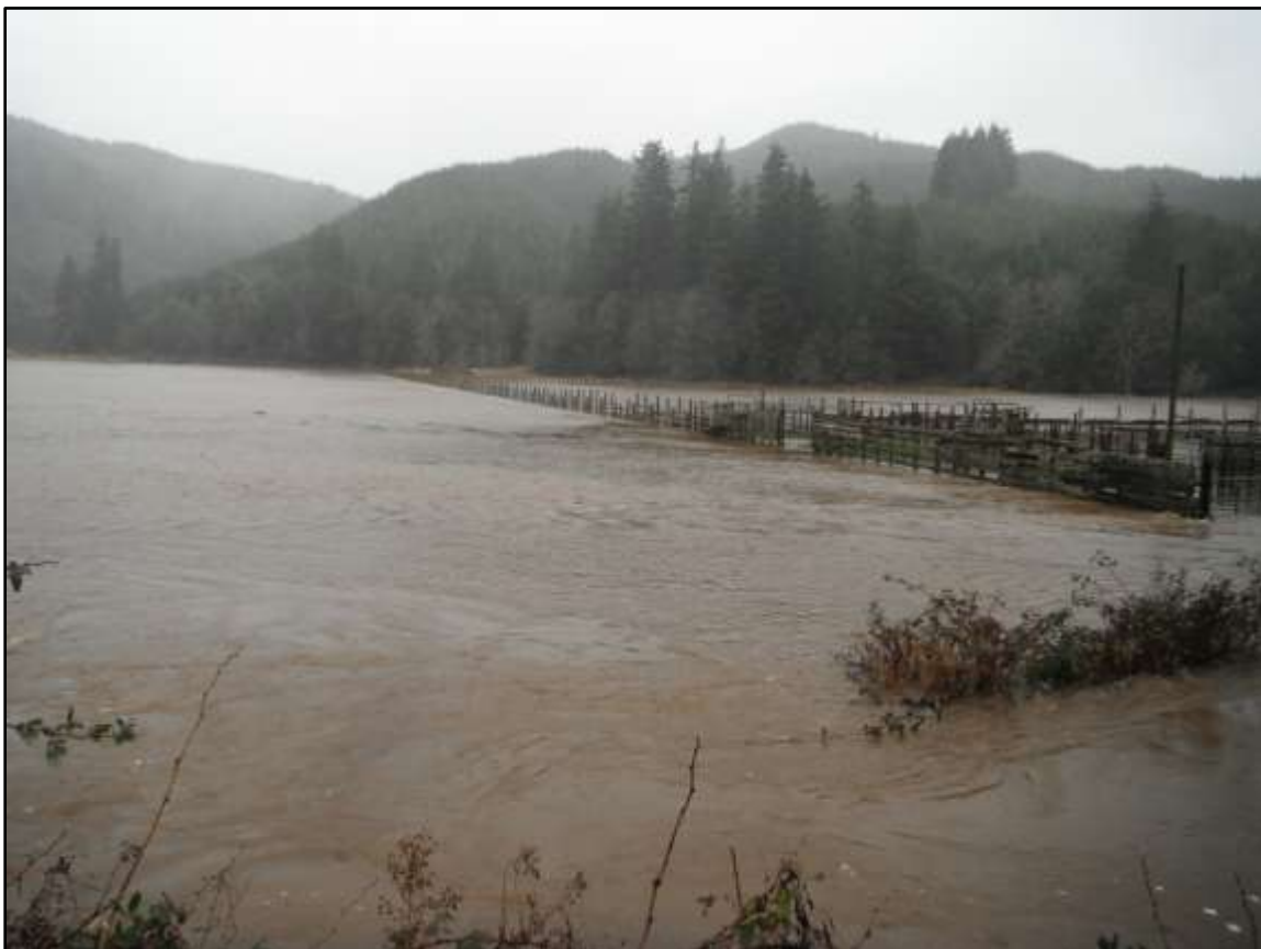
Fritz Bridge #3 is on the far side of this field. (Jan 19, 2012) Severe flooding stresses bridges in this area, but the bridge held up well.
